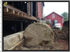
Because of its historic significance, the builders have worked with the Farm on plans to keep a portion of the cistern exposed for visitors to see. They also have resumed the repairs to the lower foundation wall. The wall repairs are progressing well; re-setting and leveling of the heavy barn stone wall is nearly complete, and new oak floor joists above the wall have been added and paired to the existing barn timbers that were in decay.
