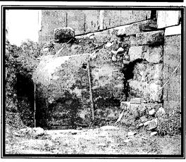
downspouts delivered water to the underground cistern. Ours is made of hand made bricks, made water tight with an exterior and interior parge coat of hydraulic cement which the farmers made themselves. It is a barrel vault design, double brick wall, about 19 feet long, 8 feet high and about 7 feet wide, it is believed to have held several thousands gallons of water. The water was piped from the cistern into the lower level of the barn to water the live stock.
